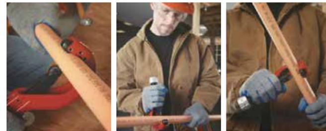
BlazeMaster pipe is easily cut with a ratchet cutter, wheel-type plastic tubing cutter, power saw, or fine-toothed saw—don't use a dull or broken cutting blade. To ensure the pipe is cut squarely, use a miter box when cutting with a hand saw. Cutting the pipe as squarely as possible provides the maximum bonding surface area.
