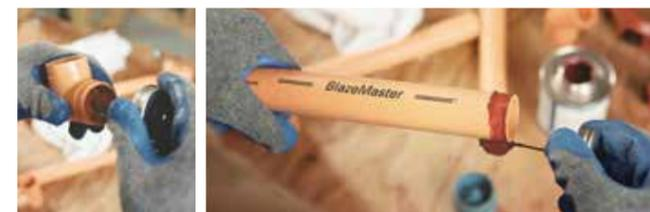
Use only BlazeMaster solvent cement which is approved for use in fire protection systems. In general, don't use solvent cement that has exceeded its shelf life or has become discolored or gelled, and don't apply solvent cement near an open flame, source of heat, or while smoking.
