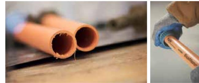
You should also create a slight bevel at the end of the pipe. This bevel helps to ease the pipe into the fitting socket without pushing the solvent cement down into the joint. For pipe sizes 50mm = 2" and larger, a complete 10 to 15° bevel is recommended.
