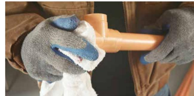
Wipe loose debris and moisture from the fitting socket and pipe end with a clean, dry rag. Moisture can slow the curing, and at this stage of assembly excessive water can reduce the joint strength.
